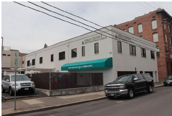
Restoration work continues in Urban Center II
