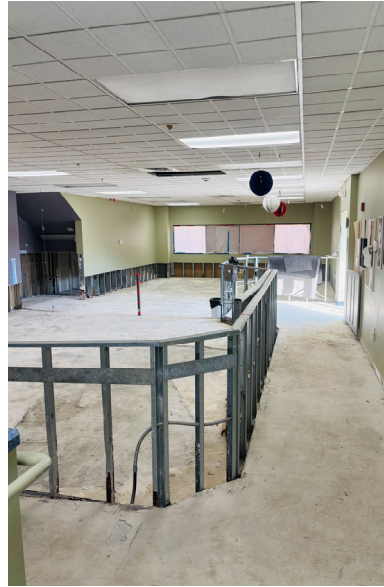
Bare flooring ready to finish
