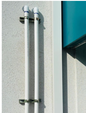
New drains installed
